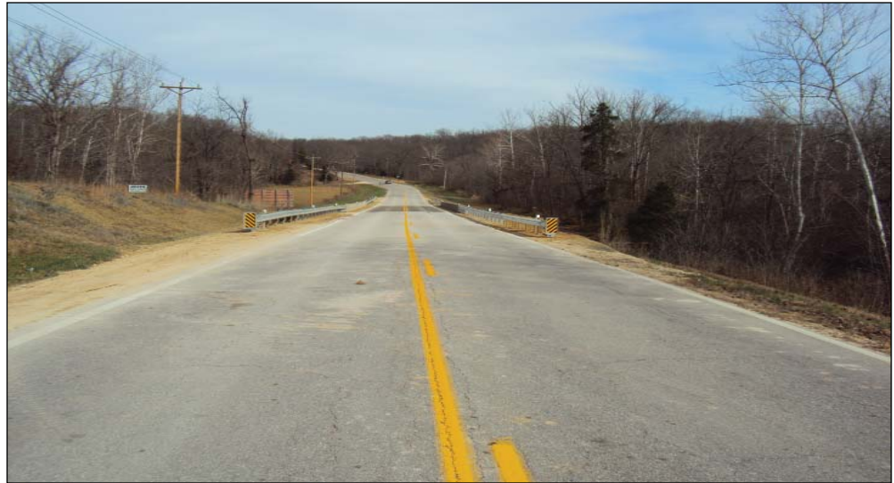
Bridge B0365 was completed on November 11, ten days ahead of an already accelerated schedule.
