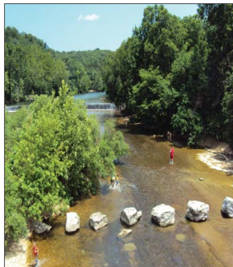
Bridge B0431 in Christian County along Route MO 125 S over Finley Creek.
