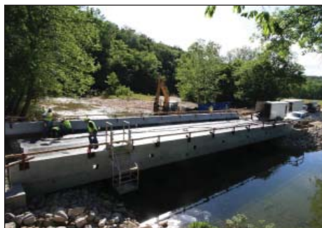
Reconstruction of the MO Route 125 Bridge over Brush Creek began May 16. Milestones included demolition of the original structure on Day 1 (top left), installation of piling on Day 2 (top middle), setting of pre-
