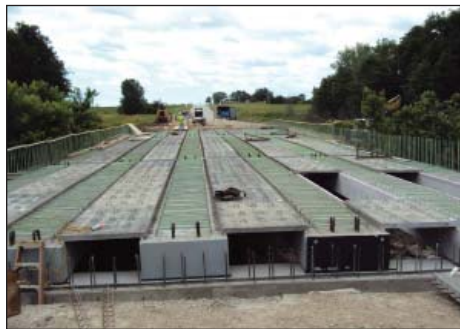
Reconstruction of the US Route 54 Bridge over the Cuivre River (top left) began June 6. Reconstruction milestones included demolition of the original structure on Day 2 (top middle), installation of piling on Day 7 (top right), pouring of end bents
