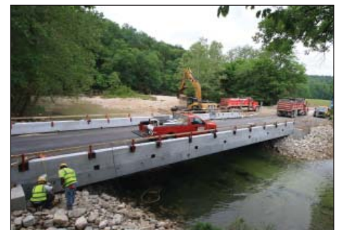
cast beams on Day 8 (top right), slipforming the barrier on Day 8 (lower left), installation of deck waterproofing on Day 10 (lower middle) and bridge completion on Day 12 – nine days ahead of schedule.
