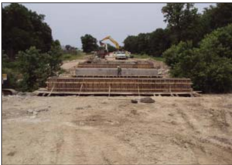
Reconstruction of the US Route 54 Bridge over the Cuivre River (top left) began June 6. Reconstruction milestones included demolition of the original structure on Day 2 (top middle), installation of piling on Day 7 (top right), pouring of end bents
