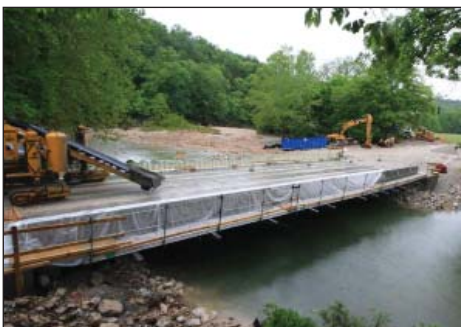
Reconstruction of the MO Route 125 Bridge over Brush Creek began May 16. Milestones included demolition of the original structure on Day 1 (top left), installation of piling on Day 2 (top middle), setting of pre-
