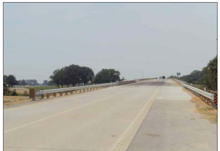
Day 7 (middle left), placing and finishing of the concrete deck on Day 18 (middle right), slipforming the barrier on Day 19 (lower left) and bridge completion on Day 22 – 40 days ahead of schedule.
